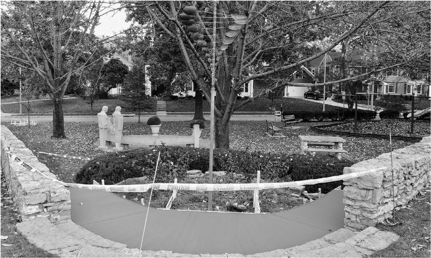
New Sidewalk & Footer Pad Poured in Preparation for Installation of New GFHA Park Sign
